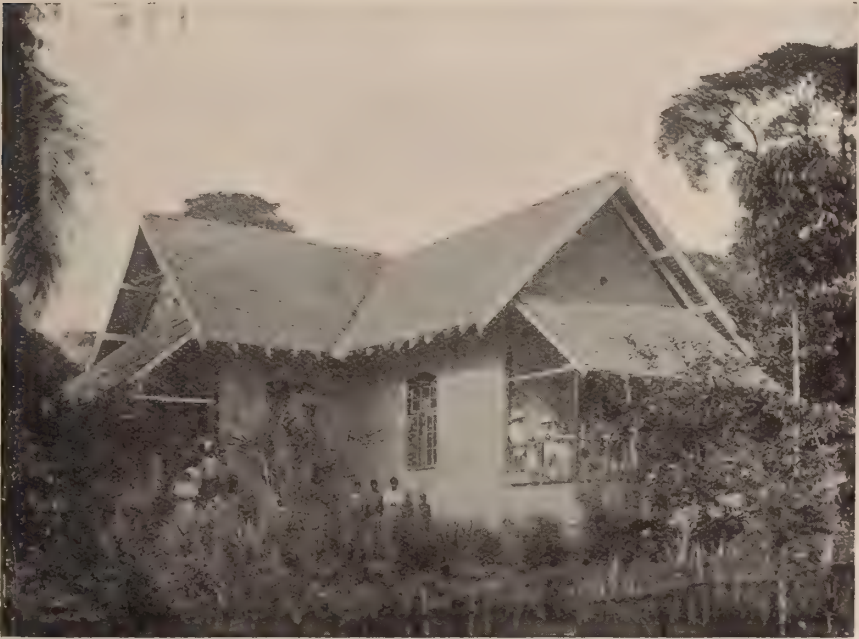
368. B.M.S. HOUSE AT BOLOBO, BUILT ON THE PLACE AT WHICH ORDEALS WERE ADMINISTERED TWENTY YEARS AGO
